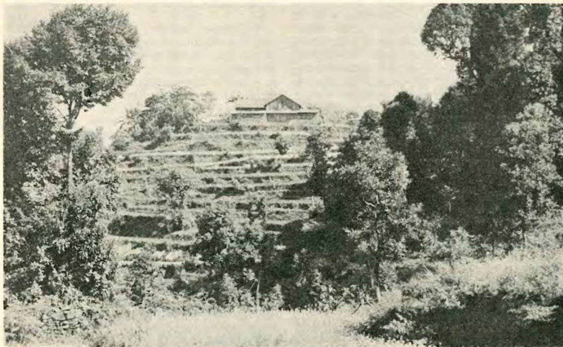
The administrative building which forms the centre of the work at Amp Pipal in the Gorkha District of Nepal. Two B.M.S. missionaries work at Amp Pipal in partnership with other missionaries and Nepali nationals.
