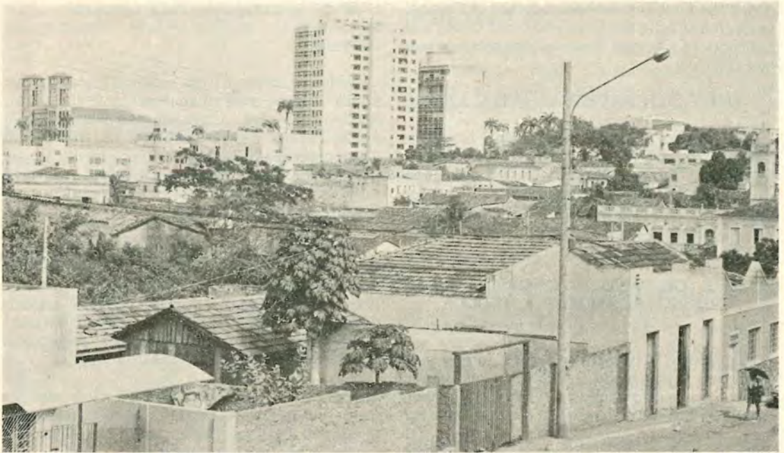
Cuiabá, centre for new B.M.S. work in Brazil.
