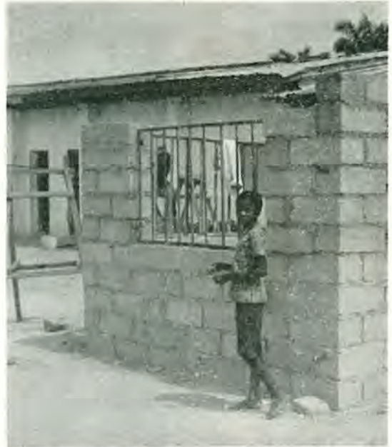
A new building at Kisangani has bars built into the windows for security.
