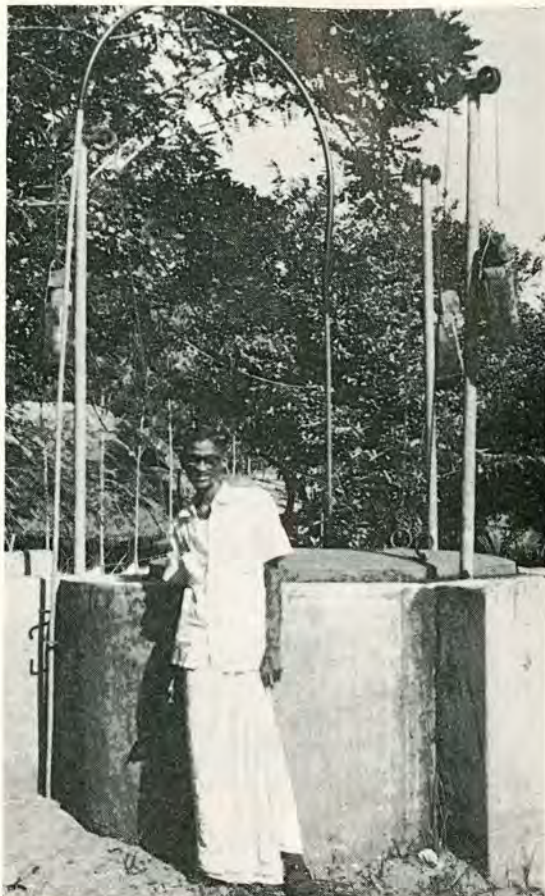
Paul, who is in charge of the New Life Centre, stands by the methane gas producer. Cattle dung is poured in daily and gas is forced from it under pressure and piped to one small gas ring which provides the cooking facilities for the Centre.
