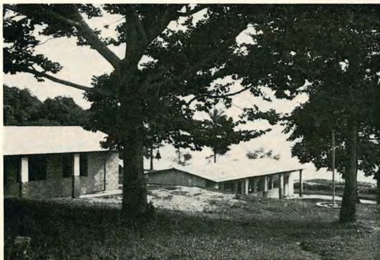
A view of some of the school buildings at Bolobo, Zaire. (Photo: D. Norkett)
