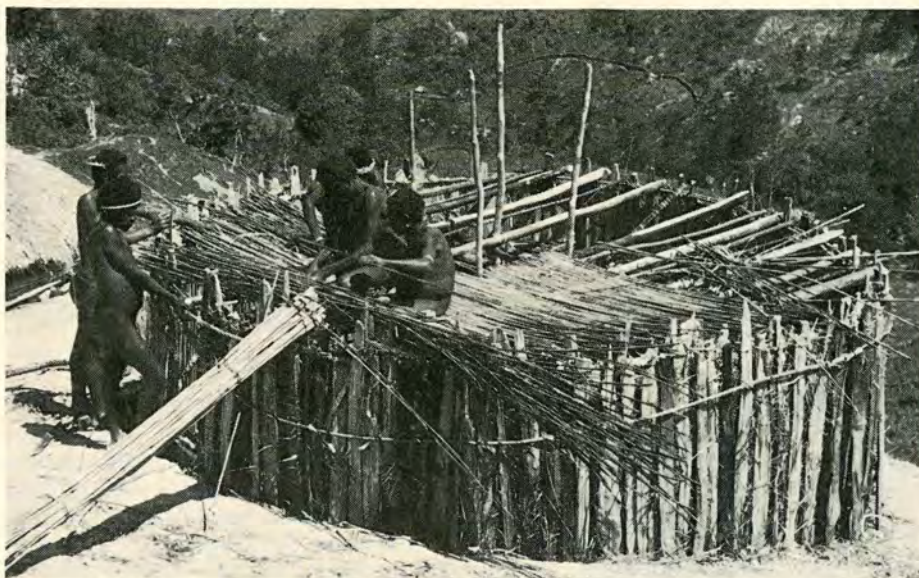
House building in Irian Jaya.
