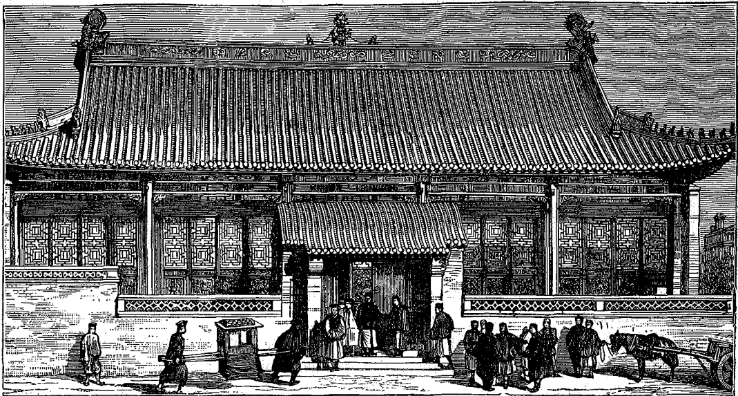
HOSPITAL AT TIEN-TSIN ERECTED BY DR. MACKENZIE.
