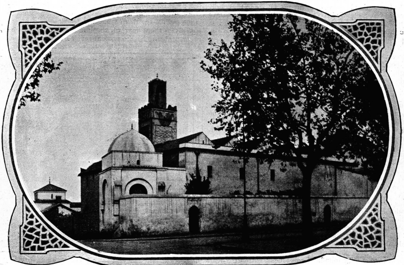
The Great Mosque, Tlemcen, Algeria.
