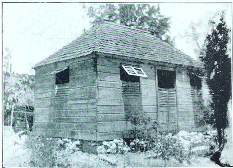
TYPICAL NEGRO FAMILY'S HOUSE, DAYRELL'S ROAD.
