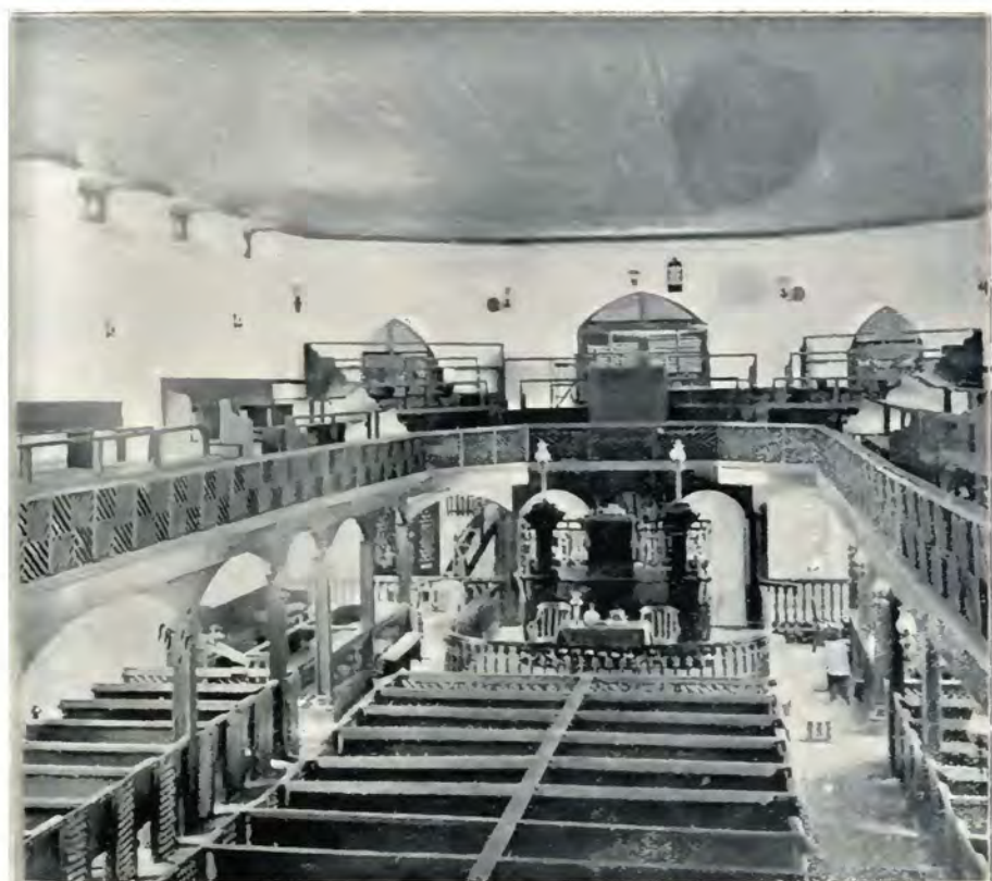
INTERIOR OF WESLEY CHURCH, CAPE COAST.
