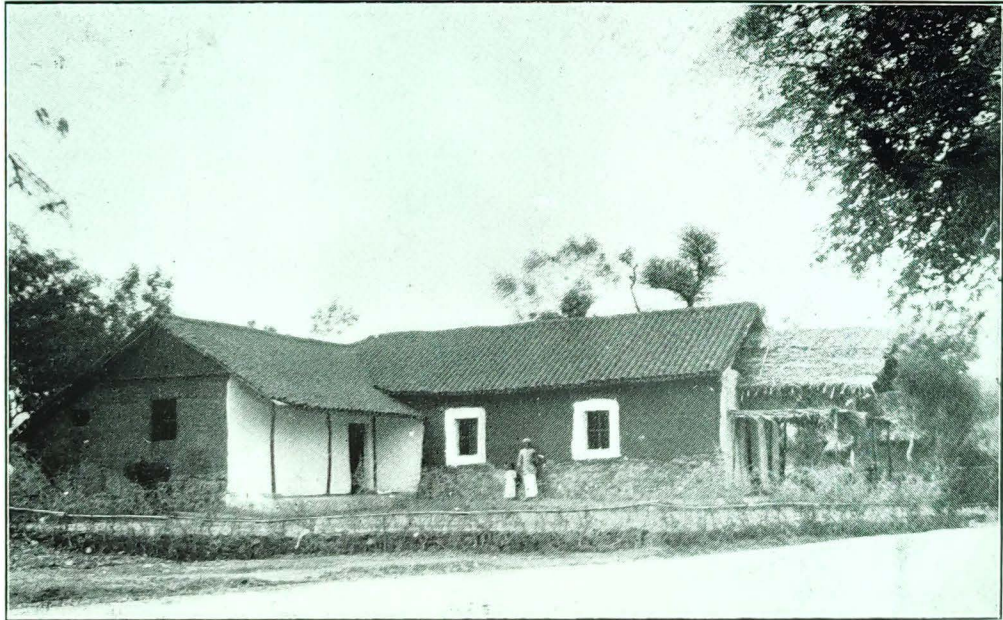
THE NEW KAKKAVERI CHAPEL (RIGHT) AND PREACHER'S HOUSE (LEFT).
